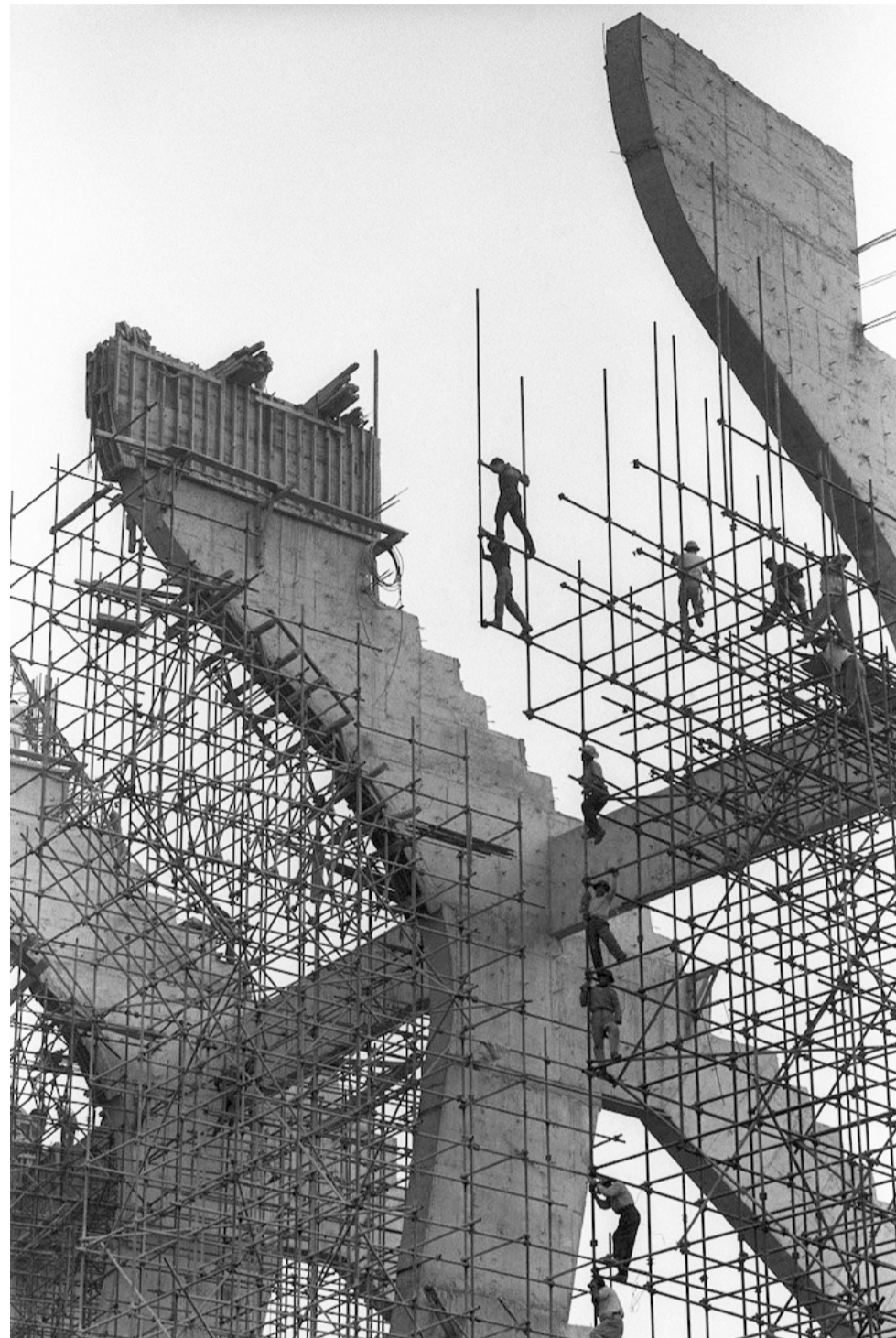
Construction of the Estadio Azteca, Mexico City, 1966
